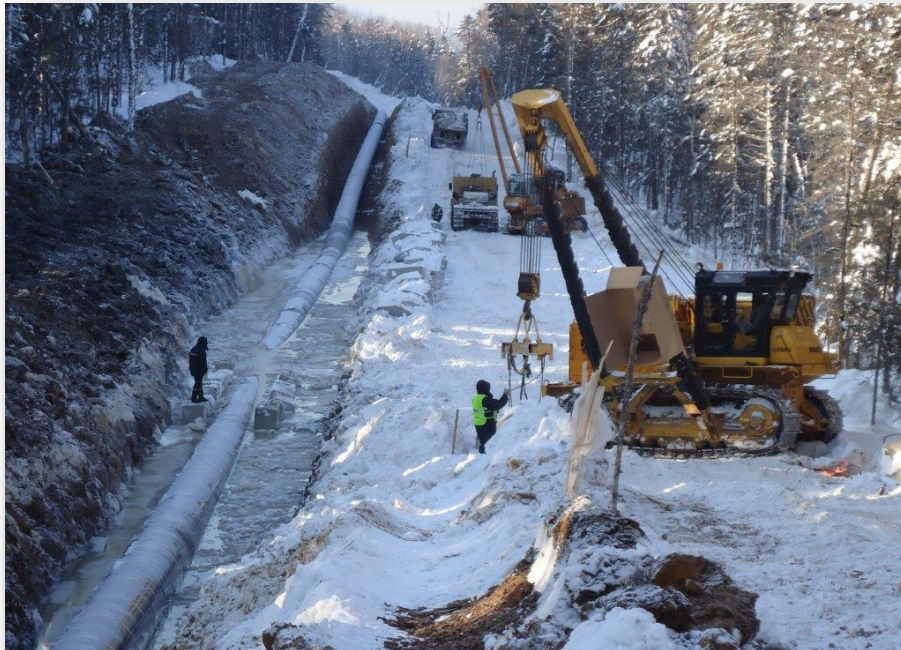
Figure 1. Pipeline construction – laying pipes in cold mountainous or rocky terrain.
